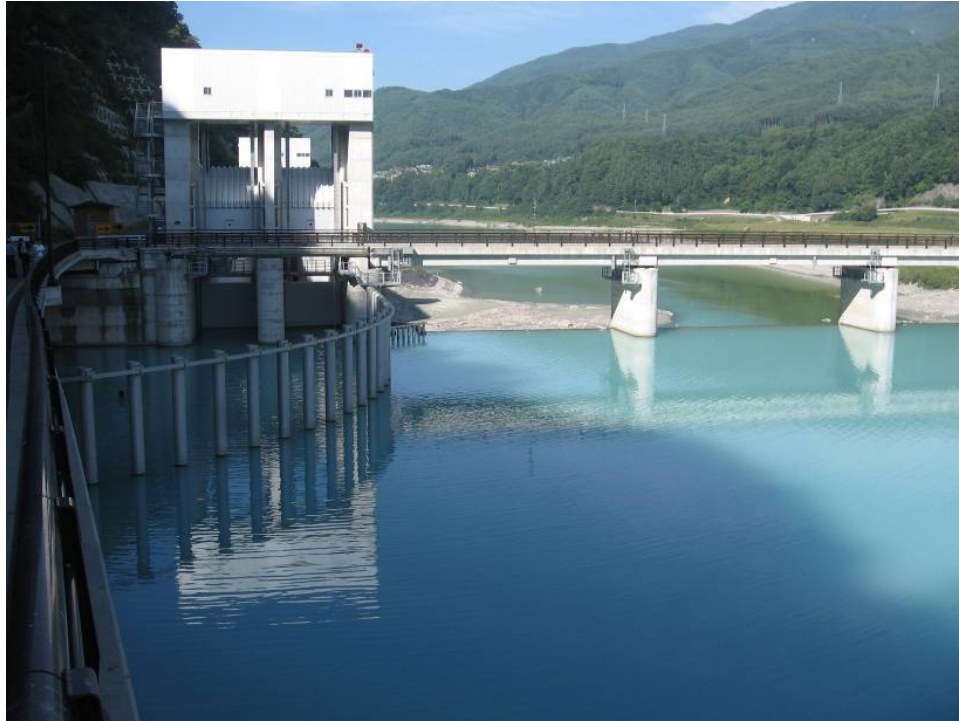
Figure 1. A diversion dam was constructed at the upstream end of the reservoir to discharge sediment laden water into the reservoir bypass tunnel. The diversion gates are on the left side of the photograph.
