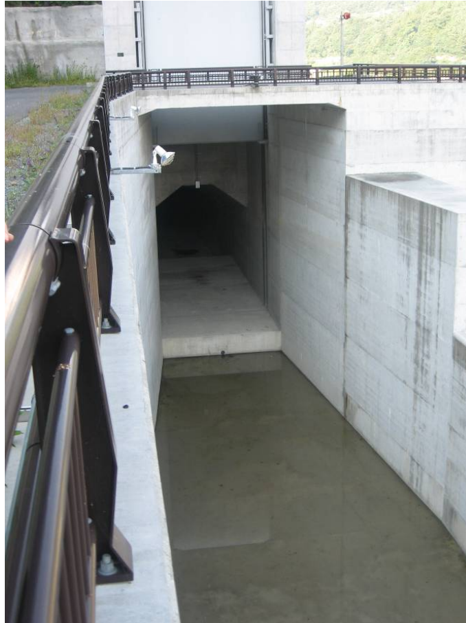
Figure 2. The sediment bypass tunnel is located at the upstream end of the reservoir and just downstream from the diversion dam.
