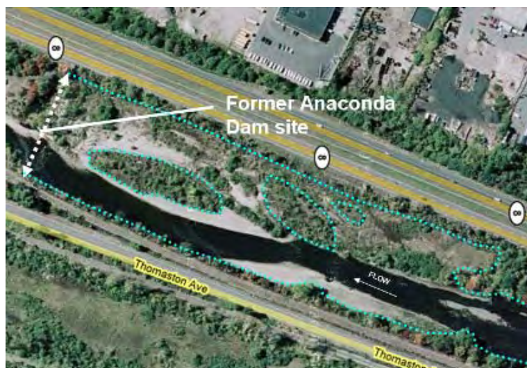
Figure 6 Anaconda Dam site 10 years post removal.
