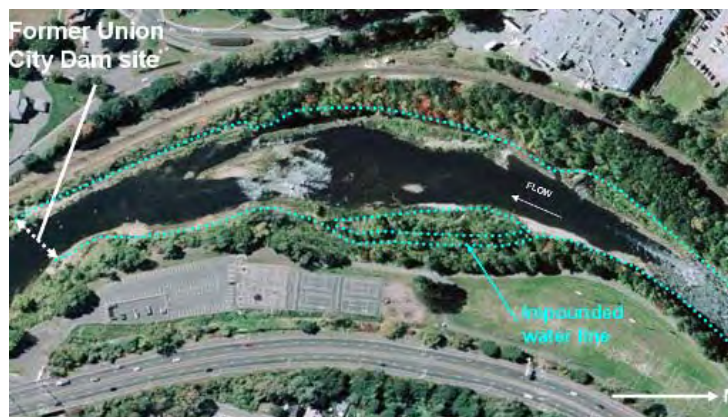
Figure 5 Union City Dam site 10 years post removal.
