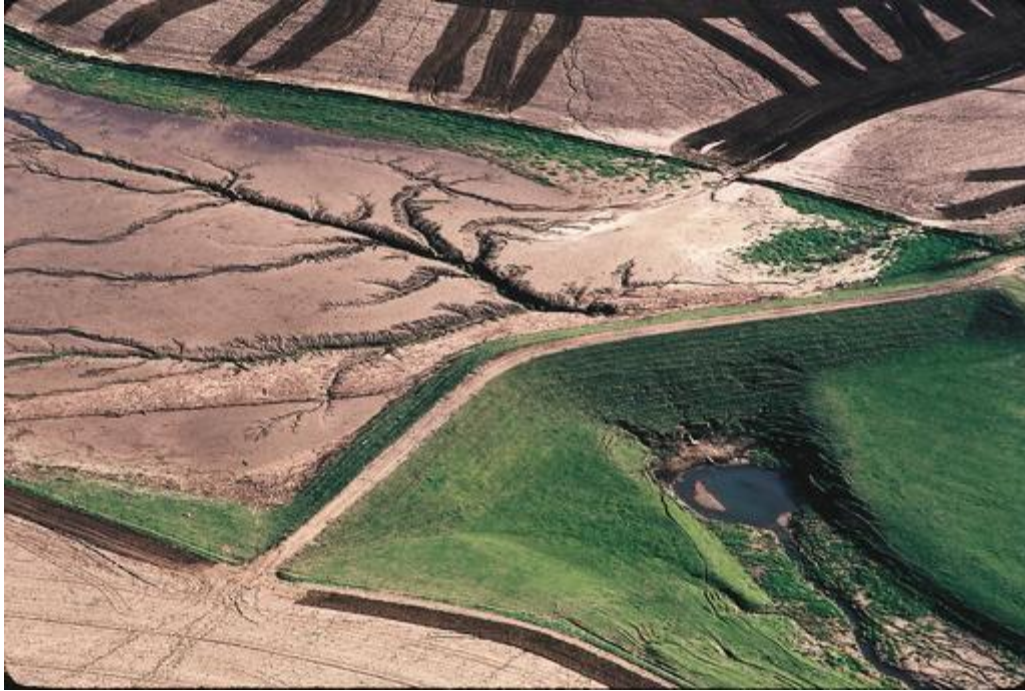
Figure 1. Dam in northwest Iowa completely silted in and no longer functioning to store floodwaters (Photo by Tim McCabe; Photo courtesy of USDA Natural Resources Conservation Service; Photo by USDA NRCS).
